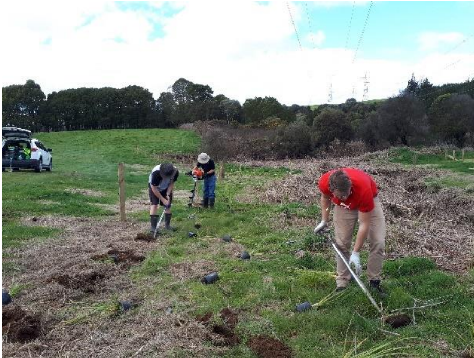
Figure 2 Gut Creek Planting and fencing
